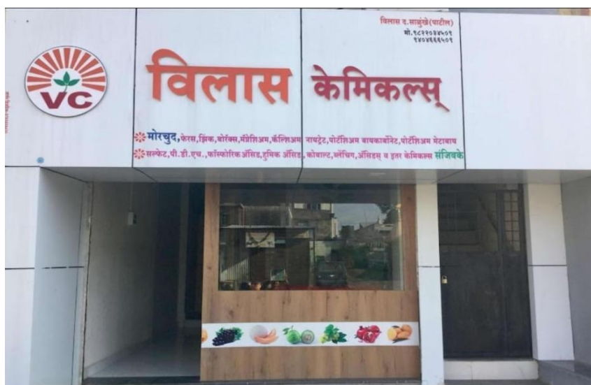
Figure 5: Vilas Chemicals - Front View of Chemical Shop, Solapur.
